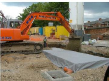
4.14 For non trafficked areas, reasonable quality as dug material is acceptable. This material however should be approved by the engineer and must not be compacted with mechanical equipment.
