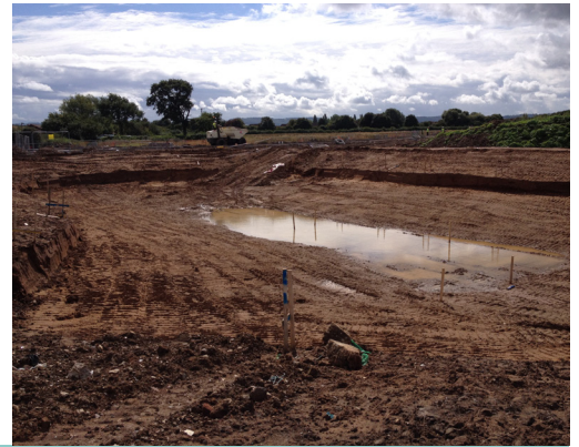
Site preparation before installation of the 1mm LLDPE
