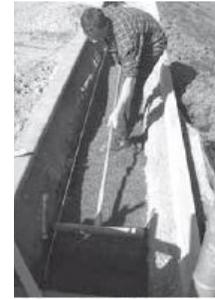
3. Lay a formation level consisting of a 30-50mm layer of 3-8mm or 2-5mm gravel. It is important the gravel contains no fines / is unbound.
