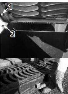
13. Fix the grating to the channel using the steel spring clips (part number DRFC008) (4 per grating) and a rubber mallet.
