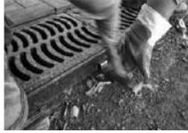
17. The Re-Medi8 media should only be placed in the channel once all paving works have been completed. Four bags of media (part number DRFC005) should be installed per every linear metre of channel. If using the 1.5m<sup>3</sup> bulk bags (part number DRFC006) of Re-Medi8, each bag contains enough media for 27 metres of channel.
