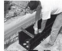
6. Lay subsequent main sections (part number DRFC001) always ensuring the pieces are properly connected to one another and free from gravel between the joints.
