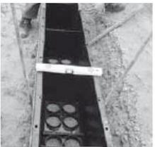
10. Now place the cast iron frame (part number DRFC007) on the D-Rainclean channel, ensuring that the location notch on the grate and the channel align correctly (1 & 2), and that each grating is placed in the same direction
