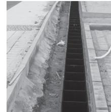
6. Lay subsequent main sections (part number DRFC001) always ensuring the pieces are properly connected to one another and free from gravel between the joints.
