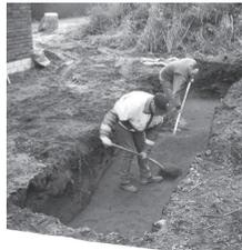
2. The top edge of the channel should be approximately 2mm lower than the finished surface level.
