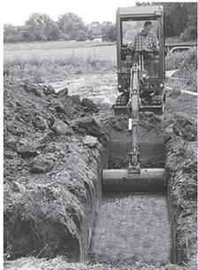
1. Excavate the soil to the required depth of the channel plus any gravel formation – see engineer's drawings. A levelling line should be laid to ensure correct alignment of the channel units.
