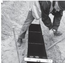
5. Lay the channel starting with an end section (part Number DRFC002), and finish each run with an end section.
