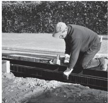
4. The difference between the formation level and finished channel level should be approximately 370mm.
