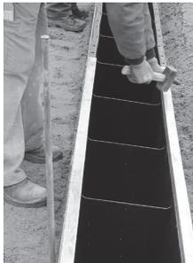
8. Where necessary the channel should be held in alignment by ground stakes or rods secured through the fixing points on the outer base edge of the channel.
