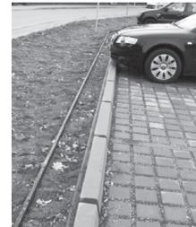
9. An end section piece (part number DRFC003) should be laid at the end of the run.
