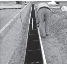
7. Ensure that the channel sections lay level on the gravel.
