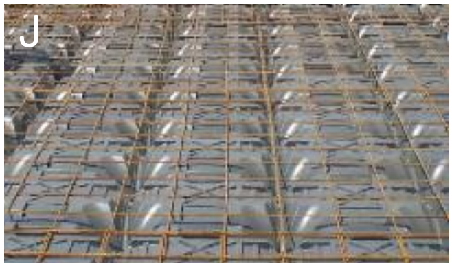
Fig J. 200mm x 200mm x 8mm of welded mesh fabric with suitable laps on top should be laid over the polypropylene forms.
