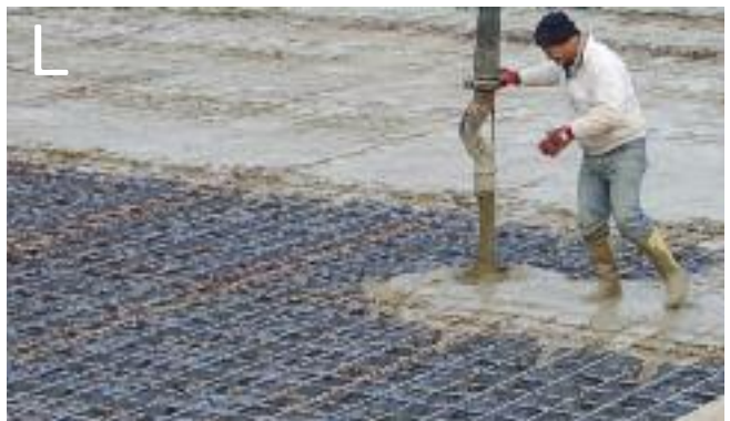
Fig L. Concrete is poured into the slab and columns to Engineer's Specification.
