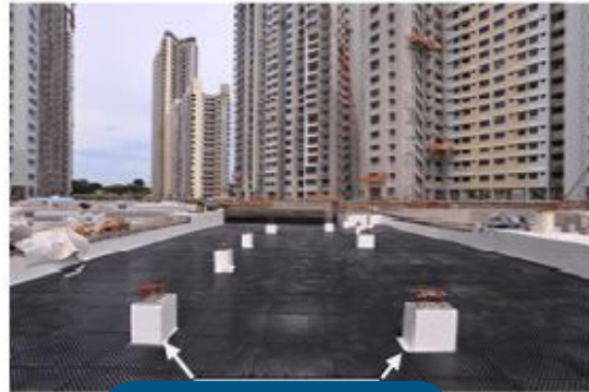
Cut to fit around plinth
