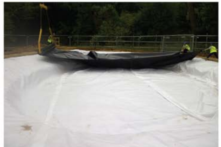
Marie Curie Pond Install, Solihull
